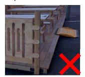
Figure 24: Ramp is used to gain access to a platform
