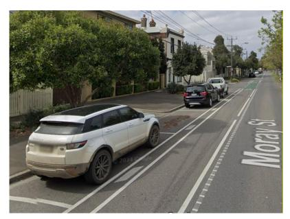
Figure 8. Moray Street, South Melbourne - buffer treatment similar to Option B
