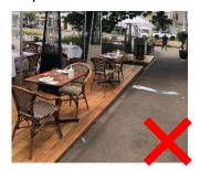
Figure 23: Platform is not flush with surround footpaths
