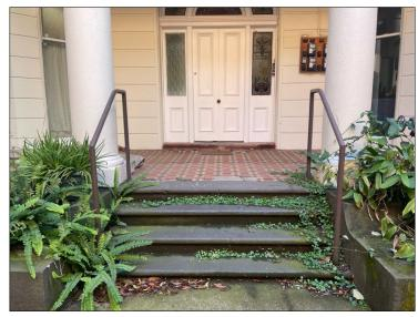
Figure 7 Front steps to the former mansion. The steps may be early or original fabric, with non-original handrails.
