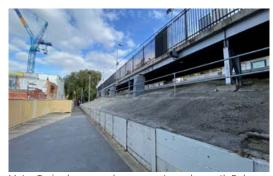
Metro Trains have used spray-crete underneath Balaclava Station platforms. Large high density housing development abutts the train station in Wilson Street
