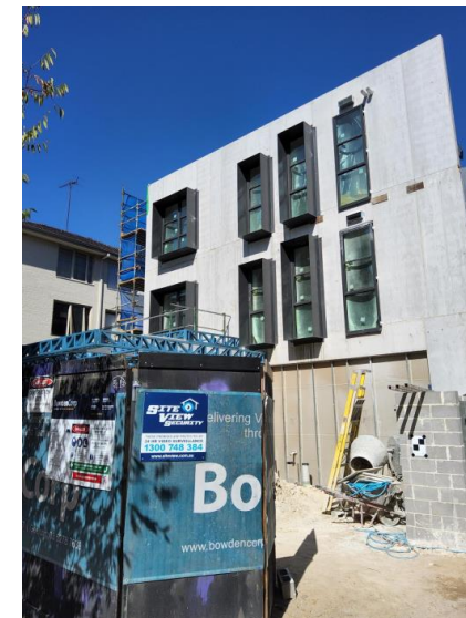
The Wellington St Ground project currently under construction (north elevation)
