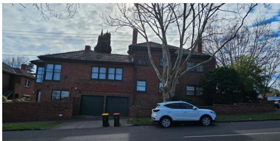
Figure 16 – South side of 18 Murchison Street to the east of the subject site. Source: Planning Officer. 4/08/2025
