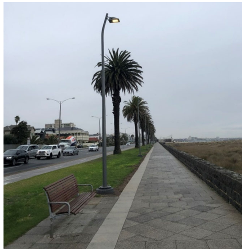
Upgraded lighting along Bay Trail
