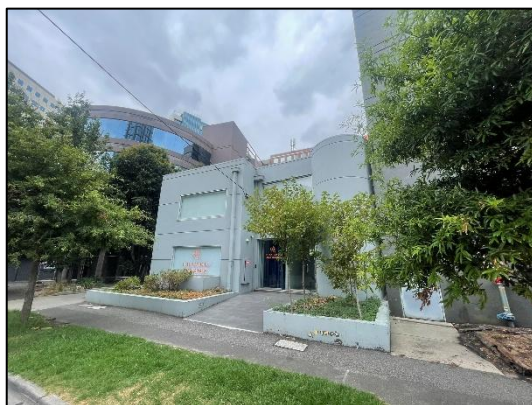
Figure 3 – Photo of the adjoining property to the north at 9-11 Palmerston Crescent taken looking east from Palmerston Crescent on 25 February 2026 (Source: Council, 2026).
