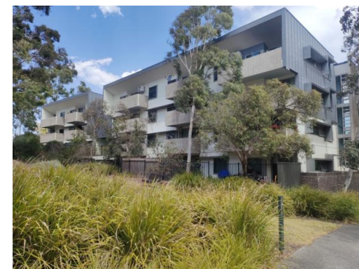
An apartment block in Port Phillip.
